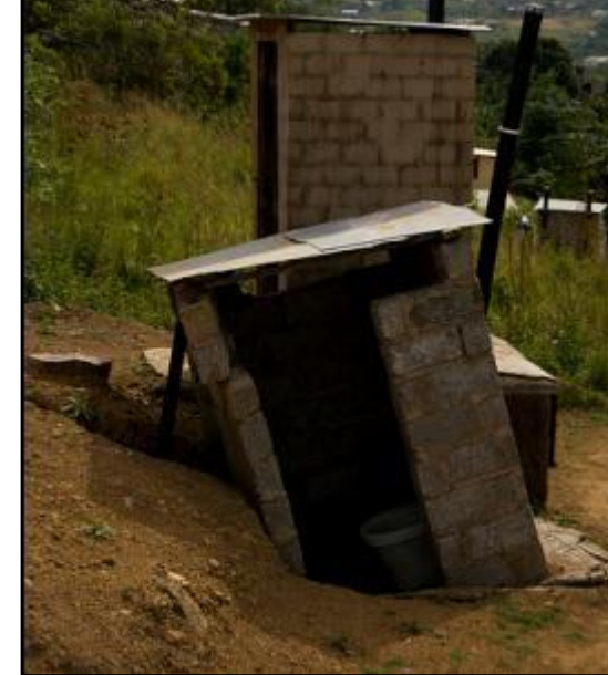
Urine diverting dry toilet (Durban, South Africa)
